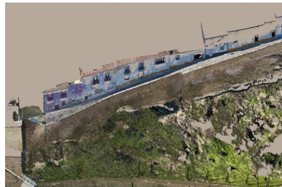
Fig. 3 Multi-source point cloud representation of the CTM section, integrating TLS and UAV photogrammetry.
